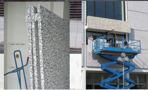
To provide a finished look during renovation, the Abteiberg Museum features lightweight panels printed on a Roland AdvancedJET to look like concrete.
